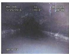
Pipe Diameter: 12" Pipe Material: Concrete?
